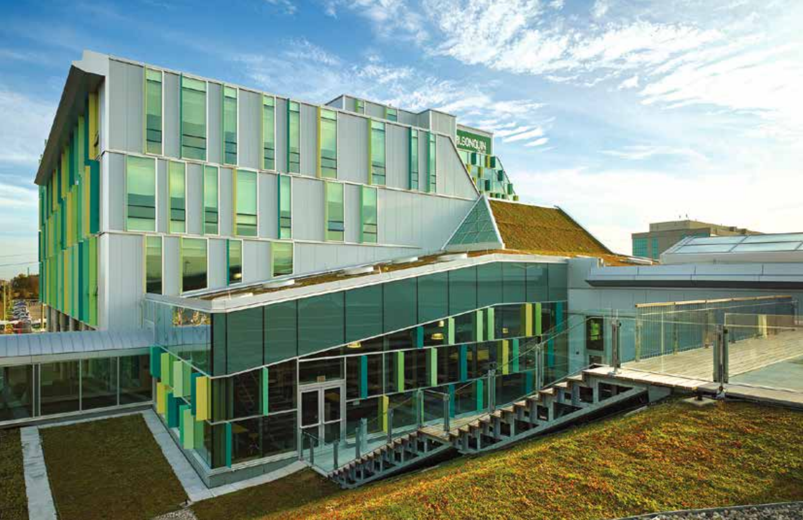
More than 85 per cent of the roof surface is covered by sedum that has self-irrigating felts, to create a broad extensive green roof.
