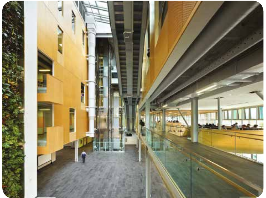
Exposed structure, ductwork, plumbing, piping and electrical services are revealed in place.
